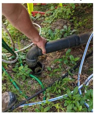
Figure 2.5 – Example Service Connection
