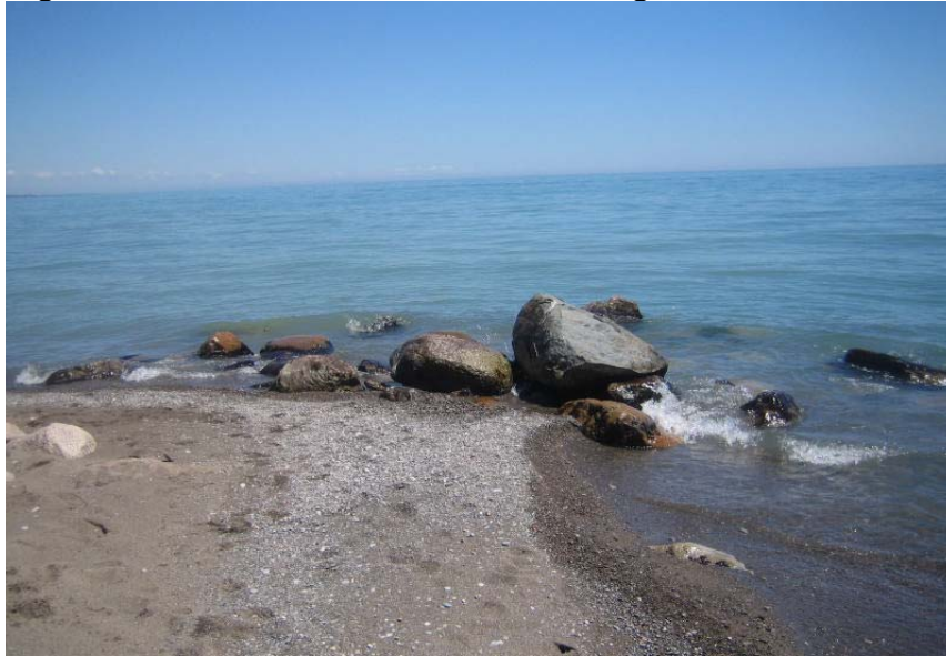
Figure 2 Field Stone Boulders Controlling Fillet Beach
